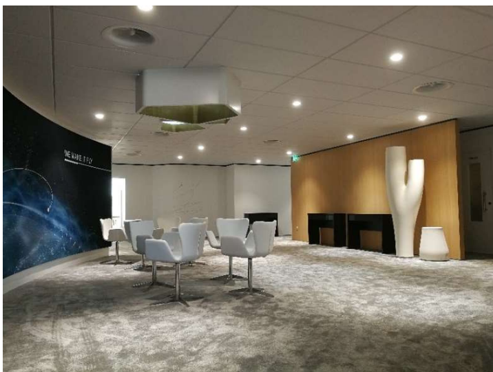
With the aid of the swirl diffusers, the ventilation technology was integrated into the Design concept.
